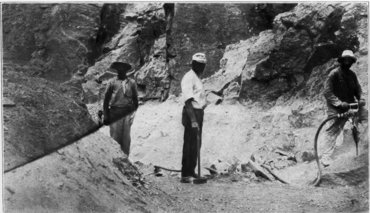
Breaking Up Large Pieces of Rock With Jack Hammer at Lewiston
